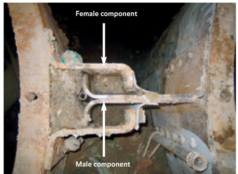
**Photo 2** Above view of the interlocking system.
