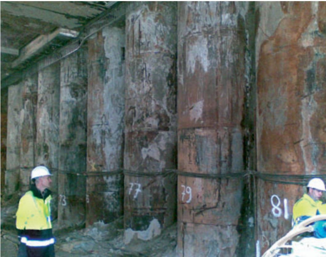
**Photo 3** View of the west MT-pile wall (excavation to NAP-6,2 m).
