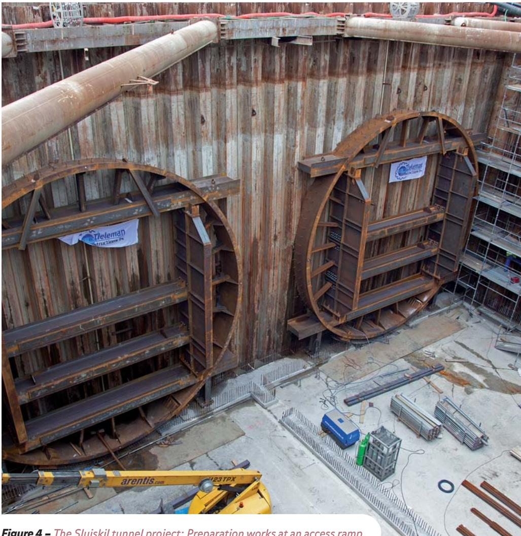
**Figure 4** – The Sluiskil tunnel project: Preparation works at an access ramp.
