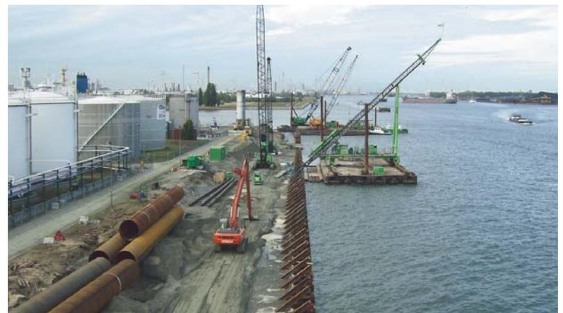
Figure 3 MV piles quay wall Antwerp (B).
