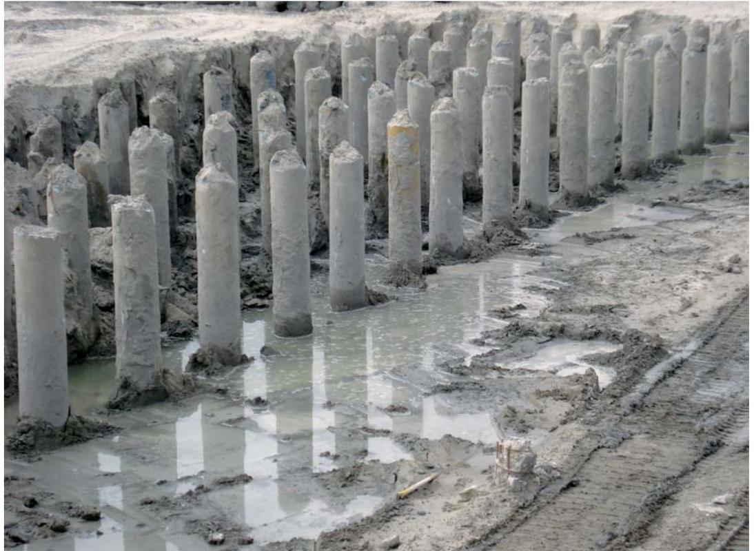
**Figure 2** Vibro-piles, installed with a noise reduction sleeve.
