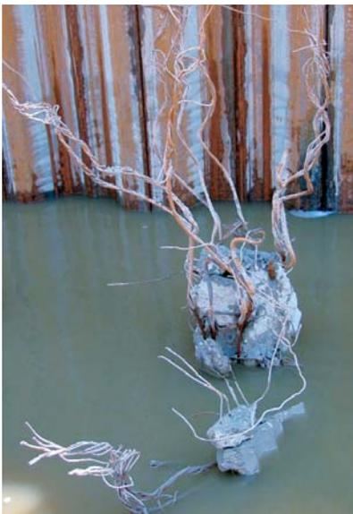
**Figure 4** Example of construction risk when driving a precast pile.
