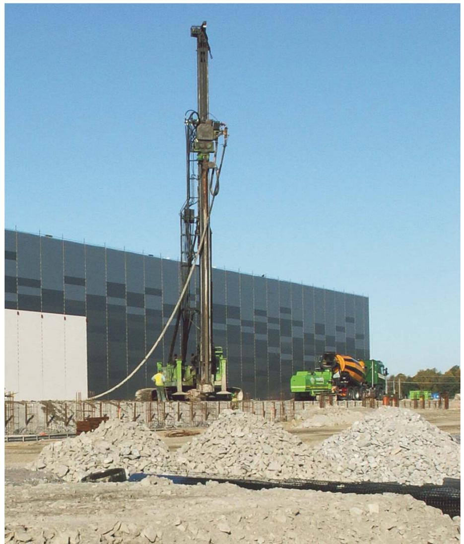
**Figure 4** The machinery used consisted of a pile crane and concrete pump. Both items are on caterpillar tracks, with relatively low ground pressure. The crane weighs some 60 tonnes. Photo: Andre de Lange, Voorbij Funderingstechniek.
