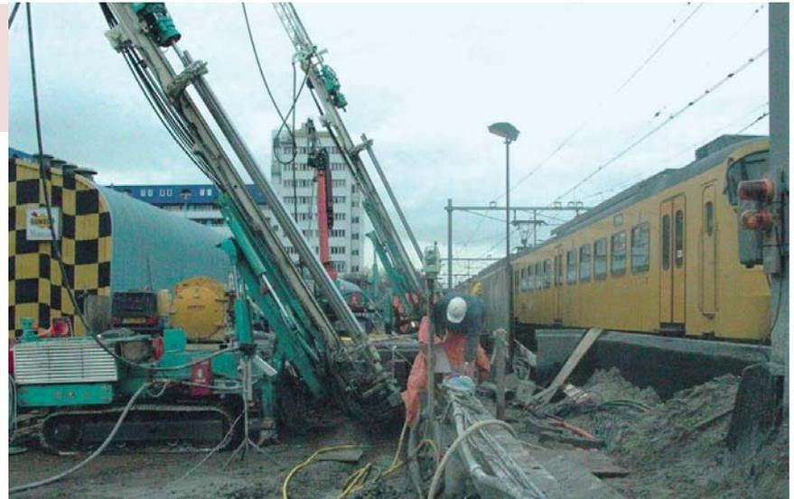
have been executed near the starting shaft. Jet grouting has been applied near the receiving shaft (figure 4). It was observed that, when realising the ground improvement techniques of jet grouting and soil deep mixing, substantial horizontal deformations occurred (several centimetres), but this did not cause any damage. However, when using these techniques in densely built areas, these deformations should be anticipated for in the design.
