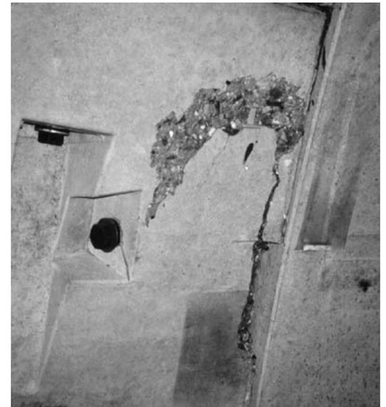
Figure 2 Damage to the Dowel and notch sockets
