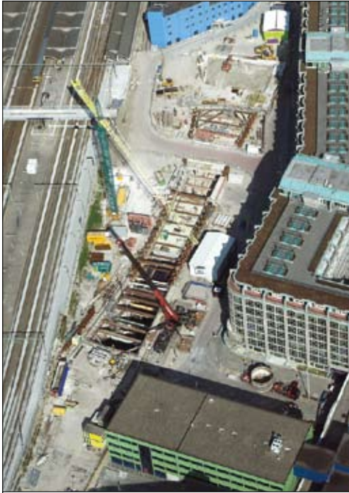
↑ Figure 3 Dismantling the TBM at the end shaft (photo Aeroview)
